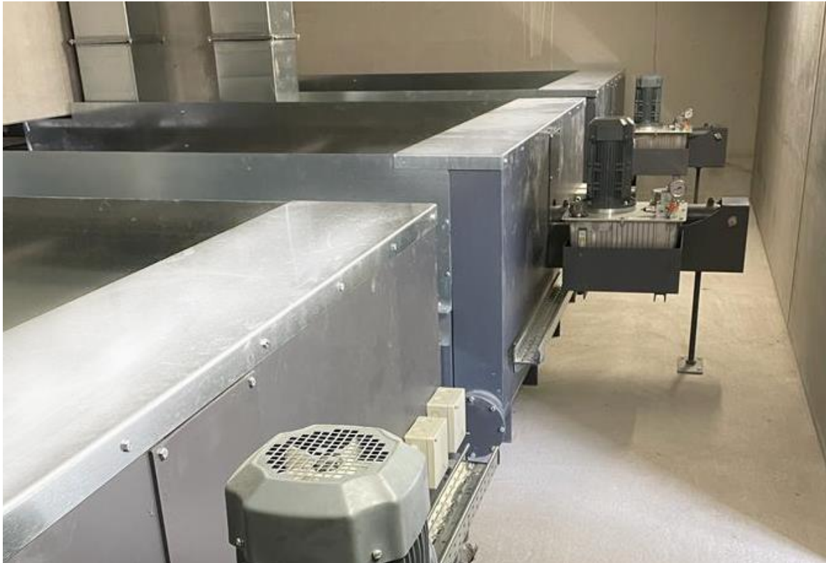
Example: Project-specific installation of three walking floor dryers.
